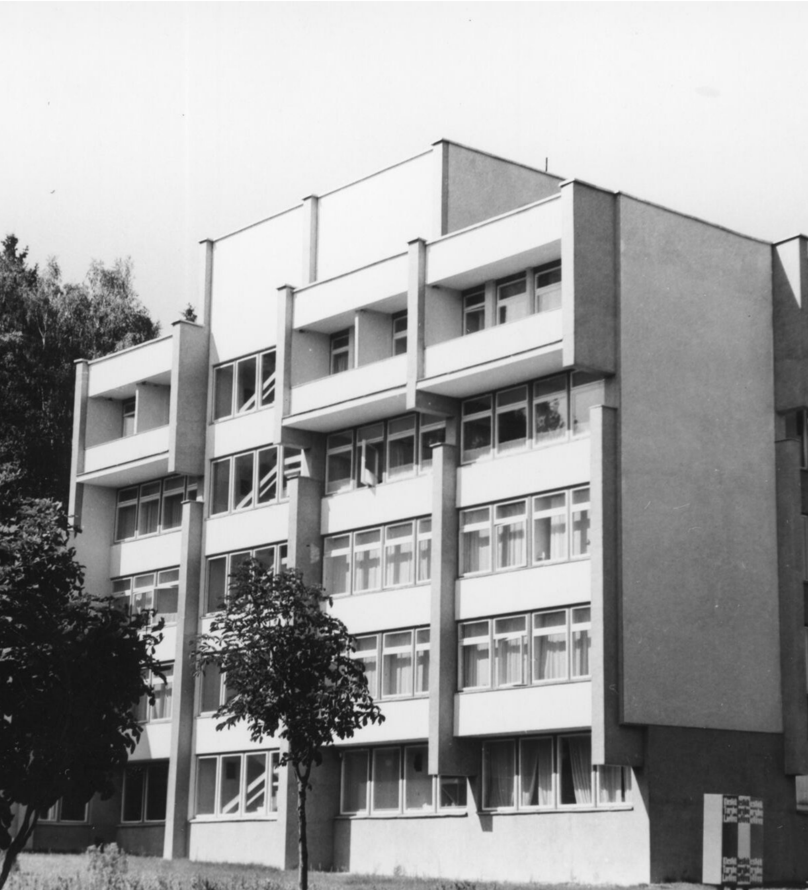
"Versmes" sanatorium administration building. Limis.lt
