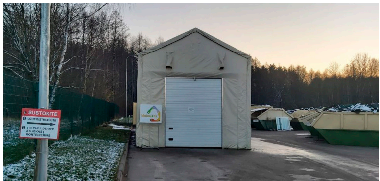
Waste sorting center
