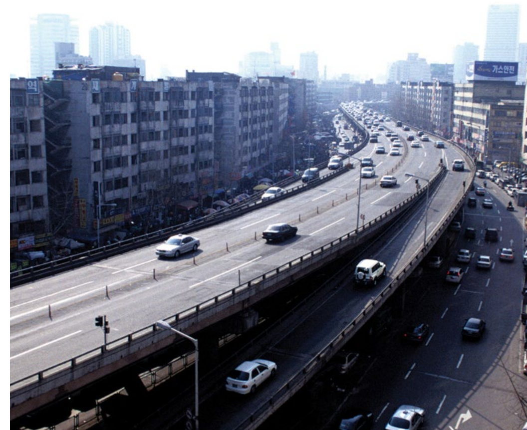
Highway before the restoration Project
